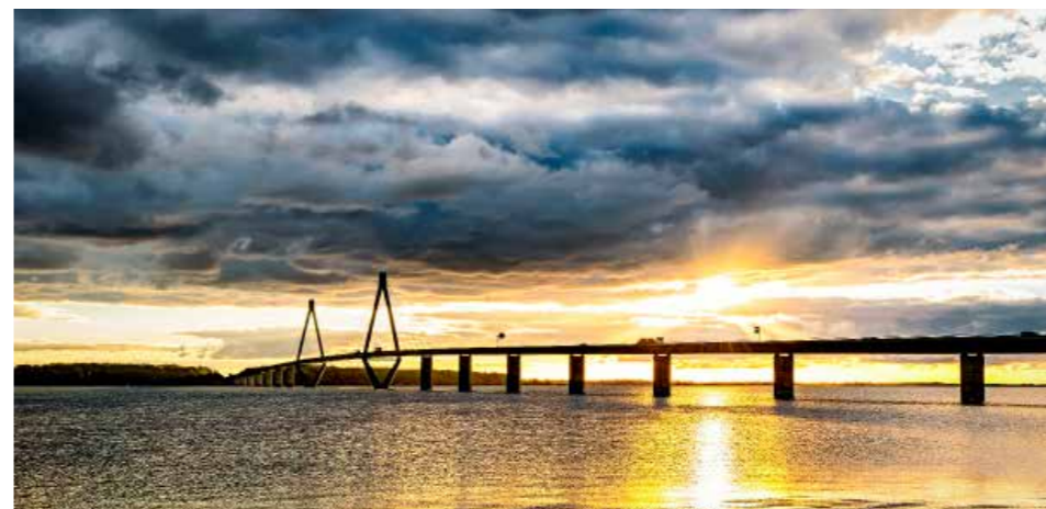
Bridge between Denmark (Copenhaguen) and Sweden (Malmö). Oresundsbron
